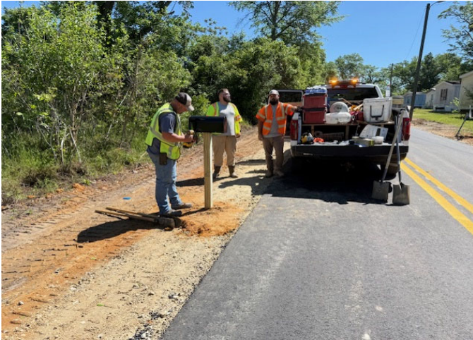
Contractor Installing Mailbox near STA 107+50 on Thomas St.
