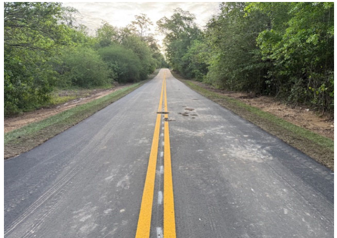
Preliminary Striping and Markers With Sod near STA 103+00 on Thomas St.
