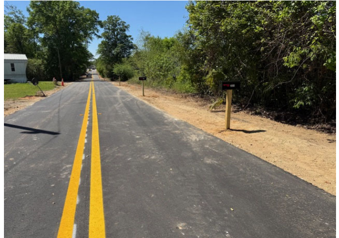
Preliminary Striping and Markers With Mailboxes near STA 108+00 on Thomas St.
