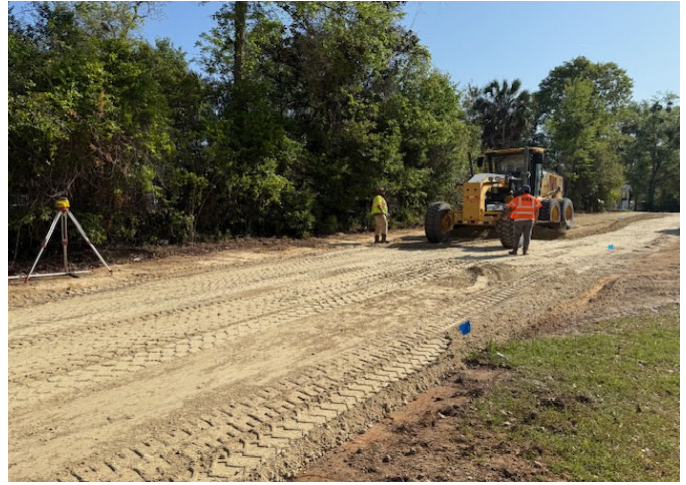
Contractor Setting Final Grade near STA 107+00 on Thomas St.
