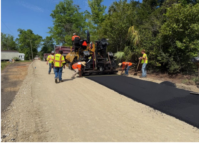
Contractor Checking Road Width During Paving near STA 109+50 on Thomas St.
