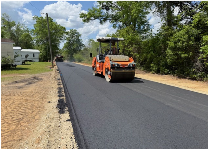
Contractor Compacting Asphalt near STA 109+00 on Thomas St.
