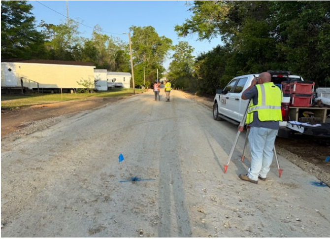
Contractor Checking Final Grade near STA 109+00 on Thomas St.
