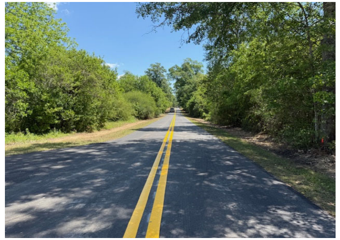
Contractor Finished Final Striping near STA 102+40 on Thomas St.
