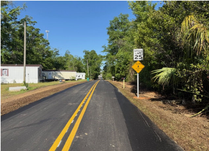
Contractor Finished Sign Installation near STA 109+60 on Thomas St.
