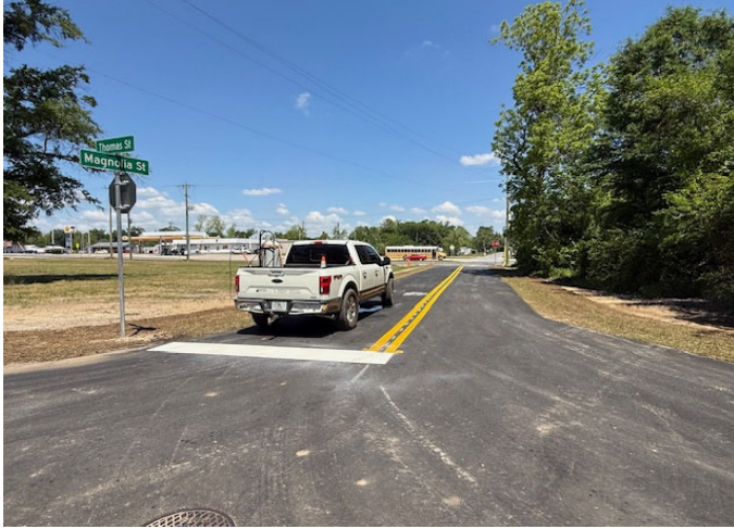
Contractor Finished Final Striping near STA 0+52 on Magnolia St.
