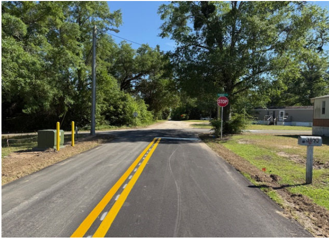
Contractor Finished Final Striping near STA 301+20 on Zion St.
