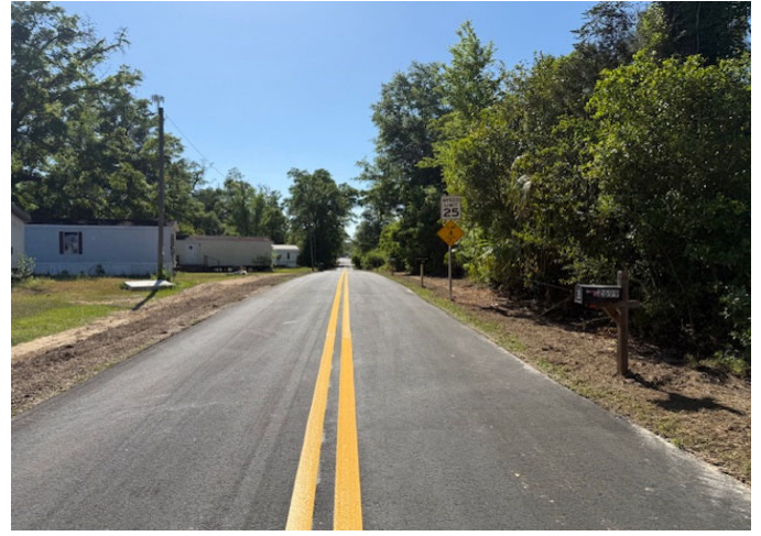
Contractor Finished Final Striping near STA 110+00 on Thomas St.
