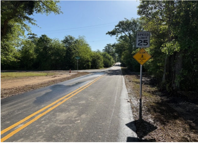
Contractor Finished Sign Installation near STA 101+17 on Thomas St. & STA 0+52 on Magnolia St.
