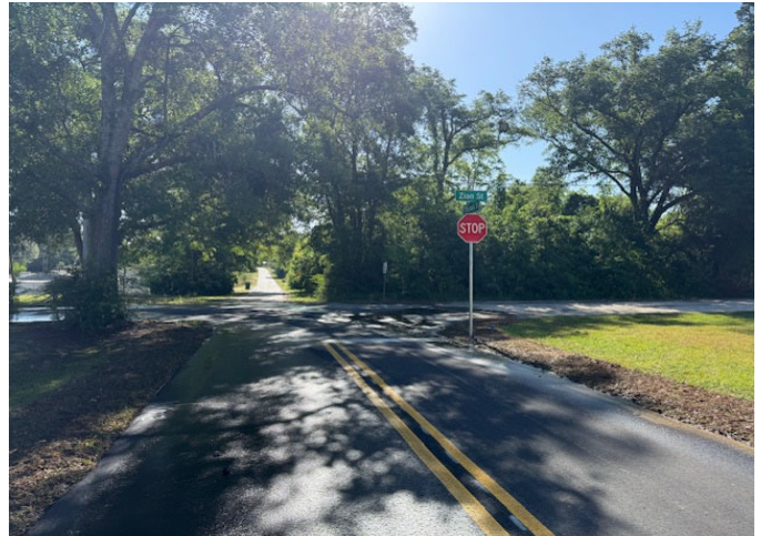
Contractor Finished Sign Installation near STA 110+70 on Thomas St.
