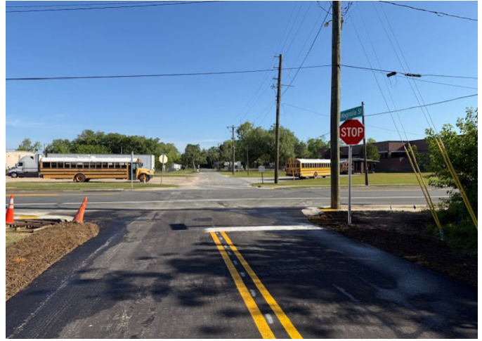
Contractor Finished Sign Installation near STA 2+05 on Magnolia St.
